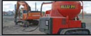
ALLU Stabilizing System Mixing of soil and a binder during stabilization process
